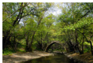
Tzelefos Bridge G00001196.jpg
